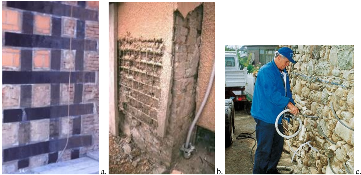
Figure 1: Examples of different methods to retrofit shear walls: a. Epoxy-bonded Carbon FRP, b. Steel mesh reinforced concrete jacketing, c. Grout Injection in the internal core of multi-leaf stone walls.
